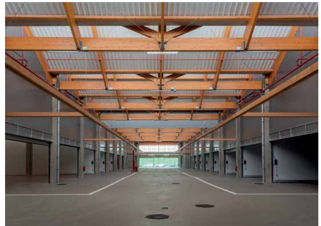
Exterior e interior del Biomarket.
